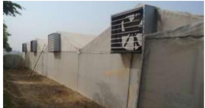
Figure 8. Co-axial exhaust fans installed in each bay of greenhouse
