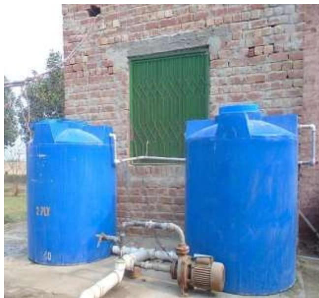
**Figure 14.** RO water storage tanks for recipe preparation
