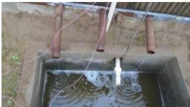
Figure 9. Drainage sump (Reservoir)
